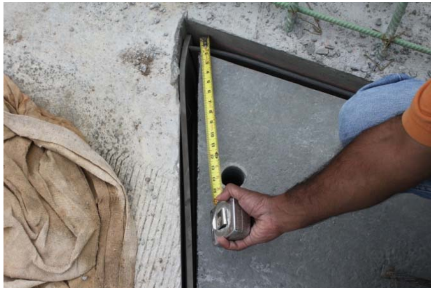
Figure 4-7 Alignment of PCPS slab with abutment
