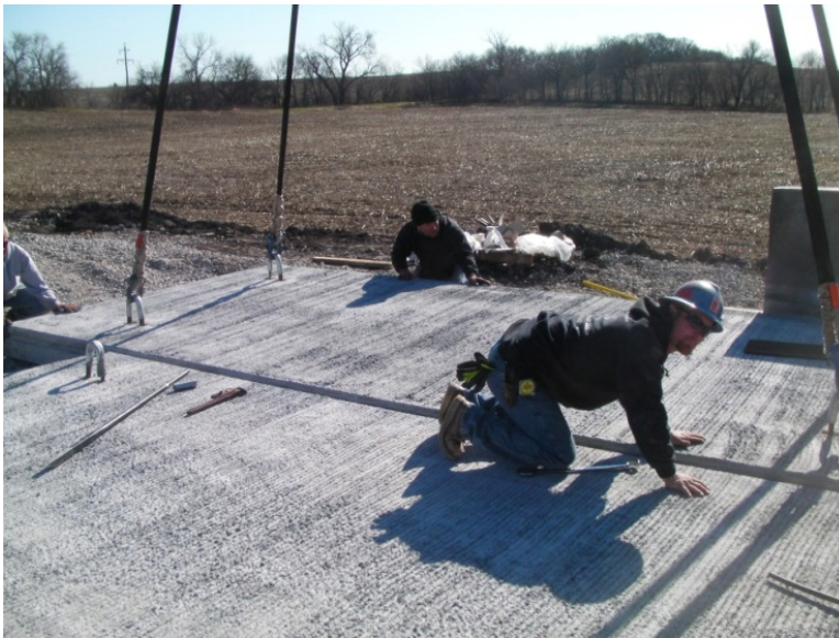
Figure 4-23 Placement of the Last PCPS Panel on Bridge A7934
