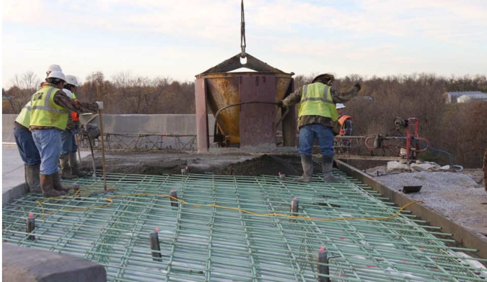
Figure 4-28 Placement of the Concrete for BAS on Bridge B0563
