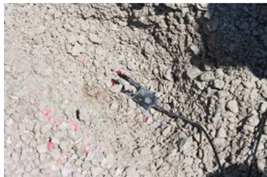
Figure 3-19 Embedding Moisture Gauges
