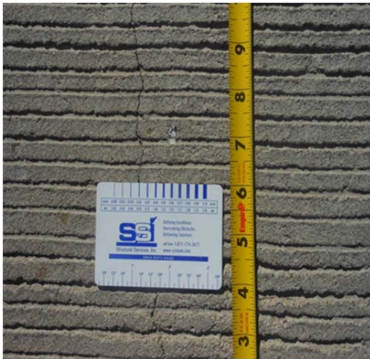
a) Measurement of crack width
