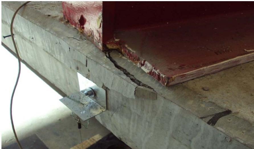
Figure 7-24 Localized Failure Due to Non-Uniform Pressure of Line Load
