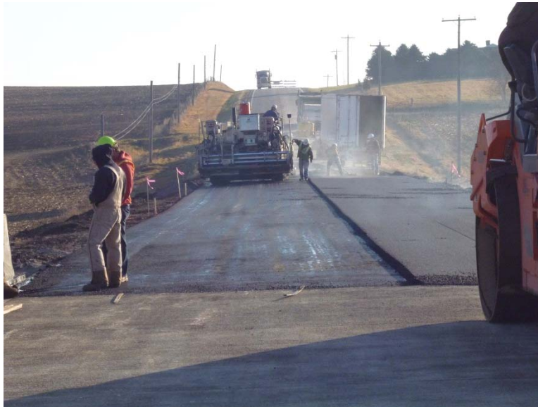
Figure 4-24 Laying of Asphalt over PCPS Panels on Bridge A7934
