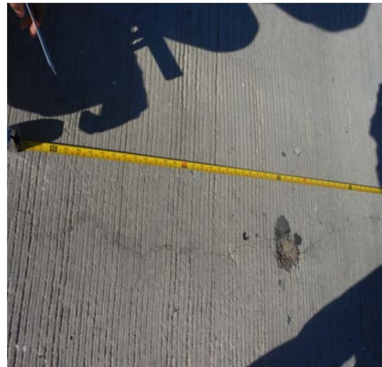
b) Measurement of crack length
