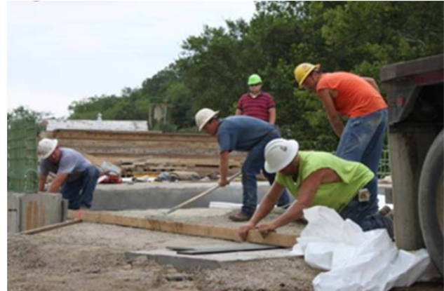
Figure 4-6 Leveling of the aggregate base
