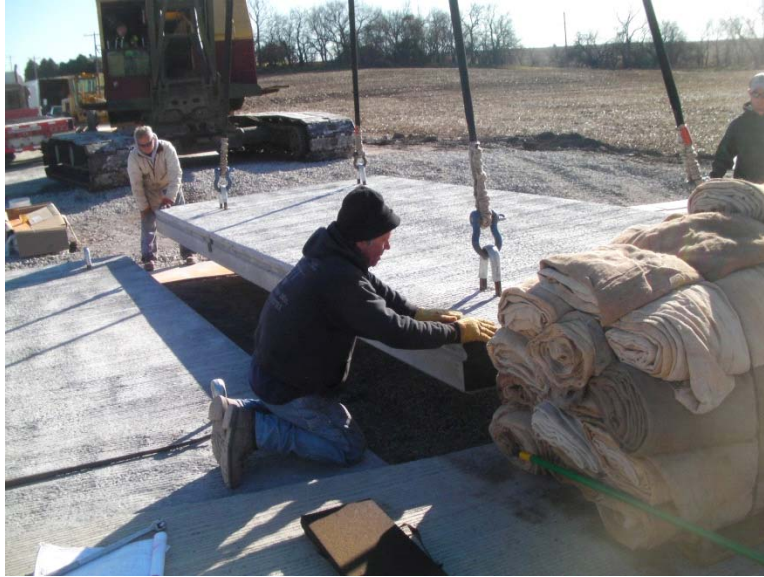
Figure 4-22 Placement of a Central PCPS Panel on Bridge on US136
