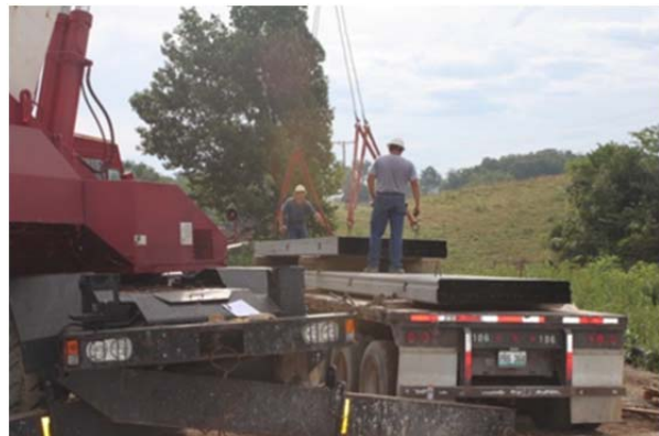
Figure 4-4 Placement of PCPS Slab Panel
