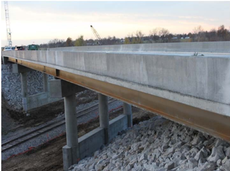
Figure 4-26 Bridge B0563 located on US71 in Barton County, MO
