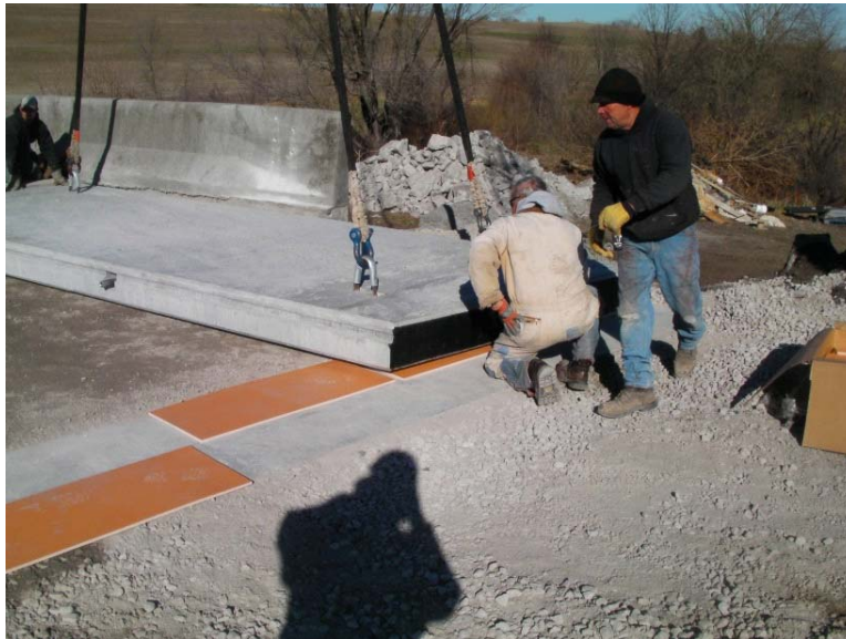
Figure 4-21 Placement of First PCPS Panel on US136 on Bearing Pads on Sleeper Slab
