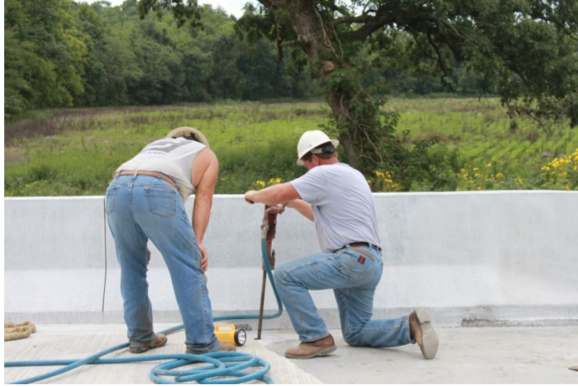
Figure 4-10 Drilling Holes in the Abutment to Connect to the BAS
