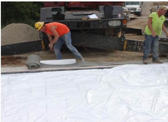
Figure 4-3 Installation of Plastic Membrane, Bearing Pads, and Joint Filler
