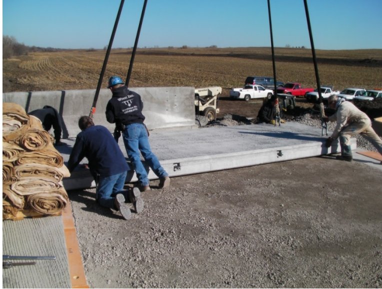
Figure 5-3 Placement of the first PCPS panel on A7934
