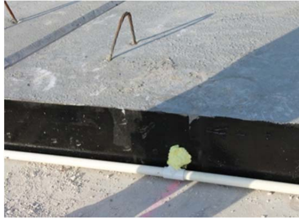
Figure 4-13 Sealing T Joints and Cable
