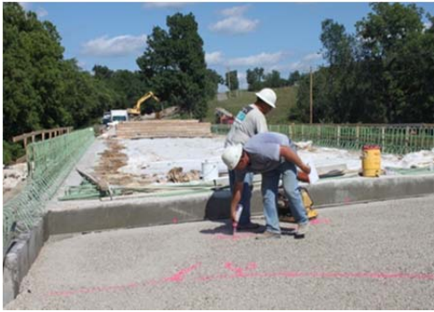
Figure 3-21 Location and Installation of the Moisture Gauges
