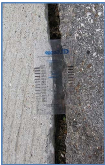
Figure 6-44 Gap between the approach pavement and approach slab at north shoulder, center & south shoulder respectively on Bridge A7890 at Final Site Inspection
