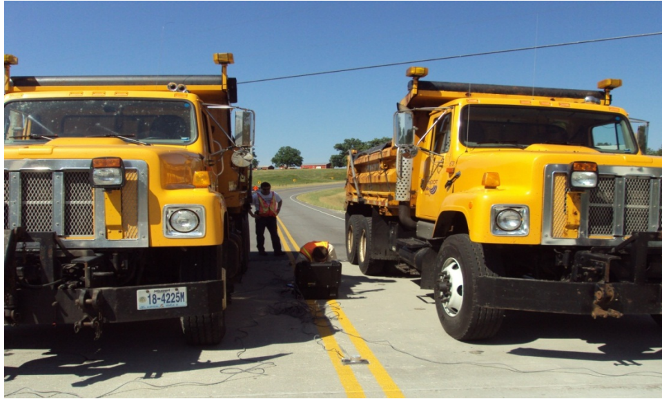
Figure 6-3 Tandem loads placed near the flexible pavement on Bridge A7890
