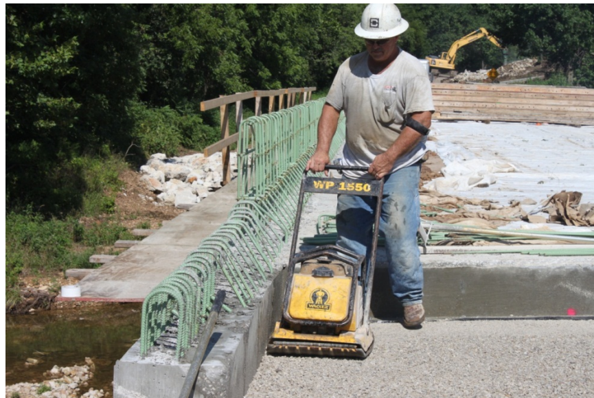
Figure 4-39 Compaction of Aggregate Base under PCPS BAS
