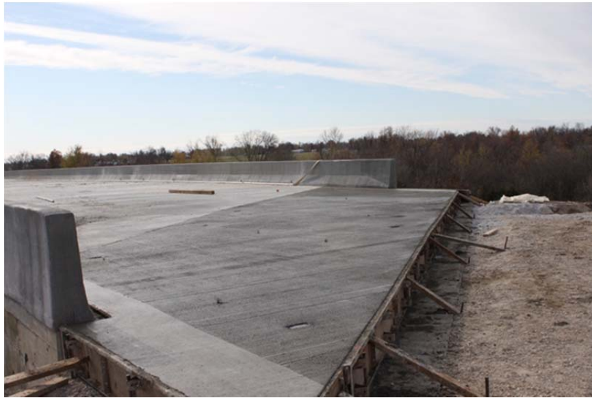
Figure 4-29 Completed Picture of 20 ft. CIP BAS on Bridge B0563
