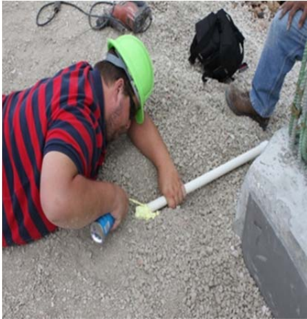
Figure 4-12 Sealing PVC Joint Conduits
