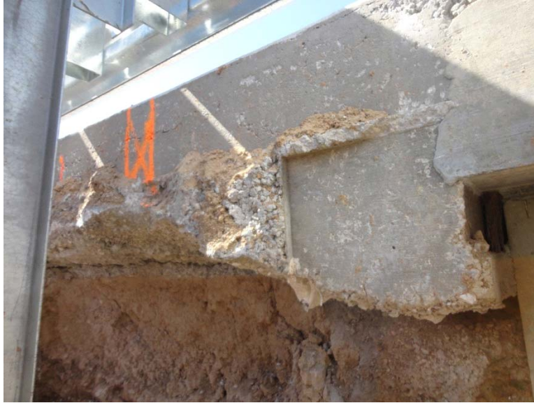
Figure 4-35 Partial Loss of Soil Support at the Edge of the BAS on the West End of MO45
