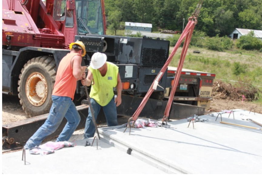
Figure 4-8 Placing the last panel
