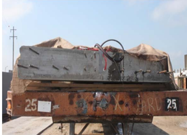
Figure 3-17 Curing of PCPS slabs
