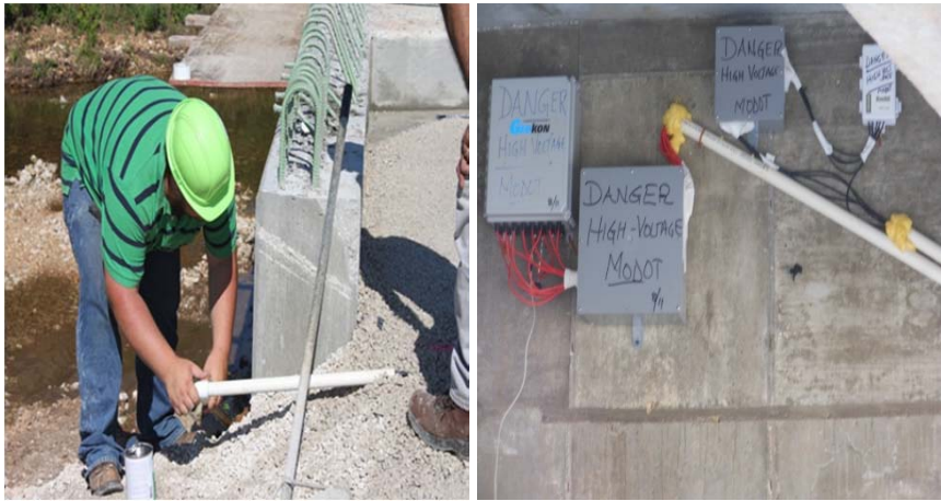
Figure 3-22 Routing Instrumentation and Data Logger Location
