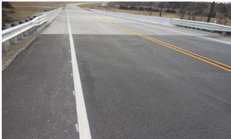
Figure 4-33 Bridge A7890 located on MO38 in Webster County, MO
