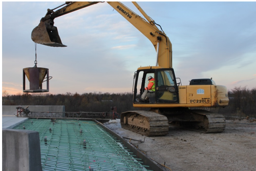
Figure 5-1 Construction of bridge B0563
