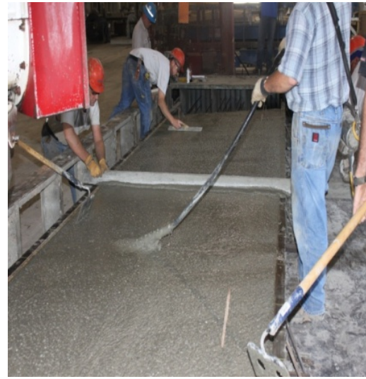
Figure 3-15 Finishing operations on PCPS slab
