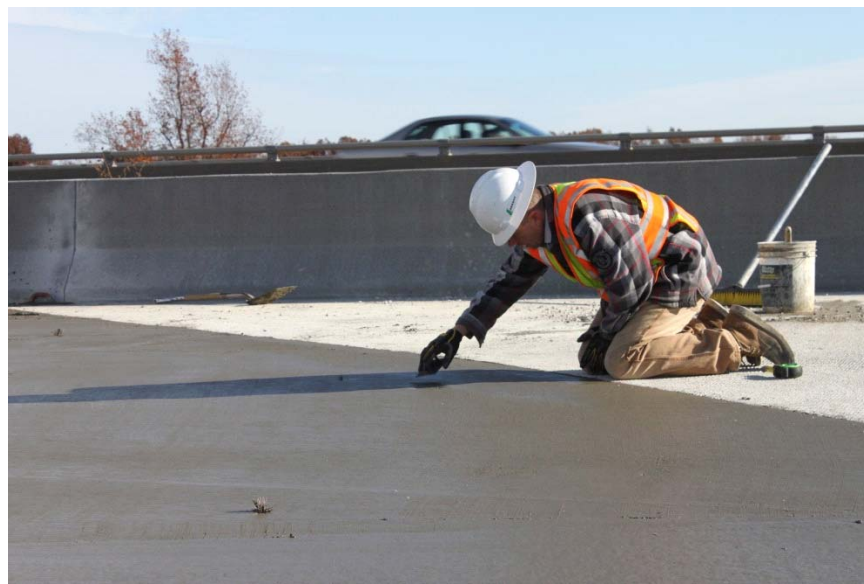
Figure 4-31 Placing Monitoring Plates Over Fresh Concrete on Bridge B0563
