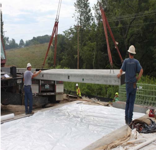
Figure 4-5 Placement of panel #1
