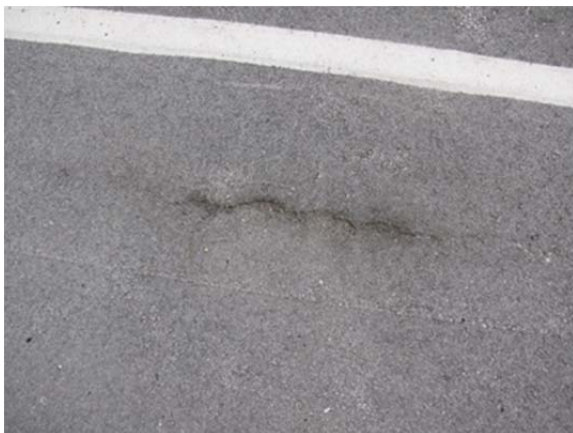
(a) Minor Longitudinal Crack
