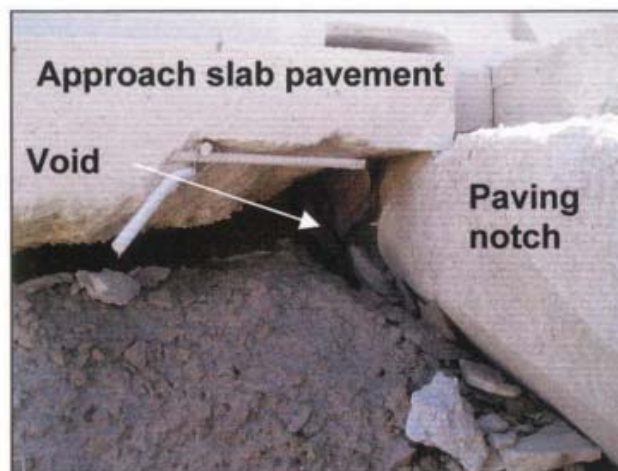
Figure 2-2 Erosion of Soil at the BAS and Abutment Joint [3]
