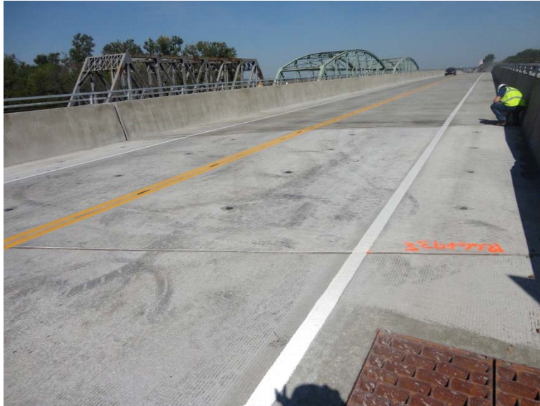
Figure 4-34 Completed View of the 25 ft. CIP BAS with No Sleeper Slab on MO45
