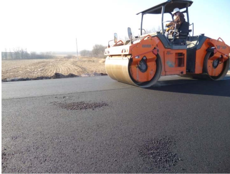
Figure 4-25 Completed Picture of the PCPS BAS system over US136
