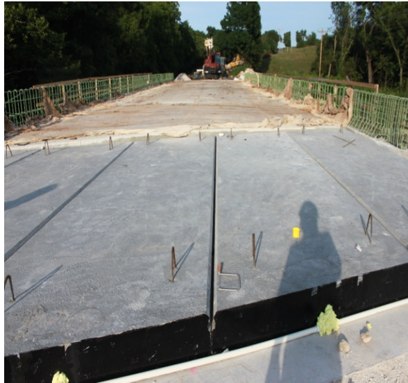
Figure 4-11 Completed Placement of All 5 Panels
