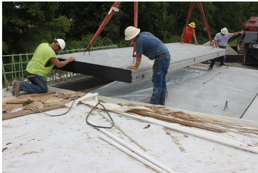
Figure 5-2 PCPS Panel placement on Bridge A7767
