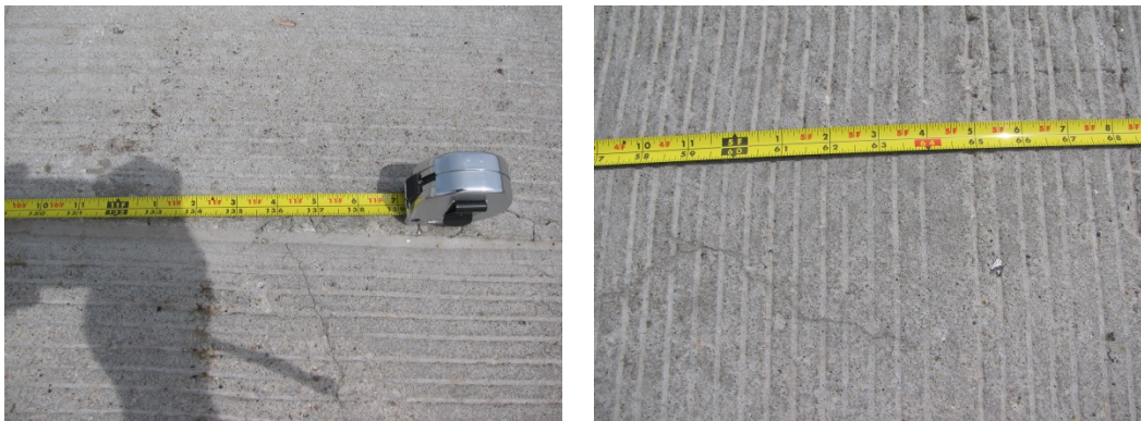
Figure 6-45 Longitudinal Crack at West End of PCPS on MO38 – 11’4” distance from the wing wall (left) and 5’4” crack (right)
