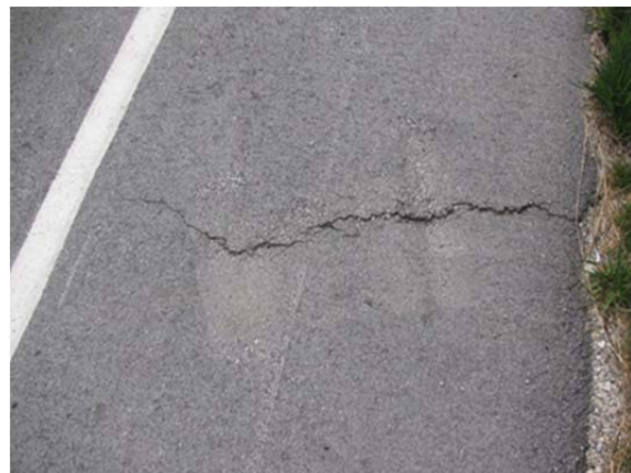
(b) Transverse Shoulder Crack
