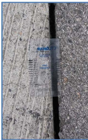
Figure 6-44 Gap between the approach pavement and approach slab at north shoulder, center & south shoulder respectively on Bridge A7890 at Final Site Inspection
