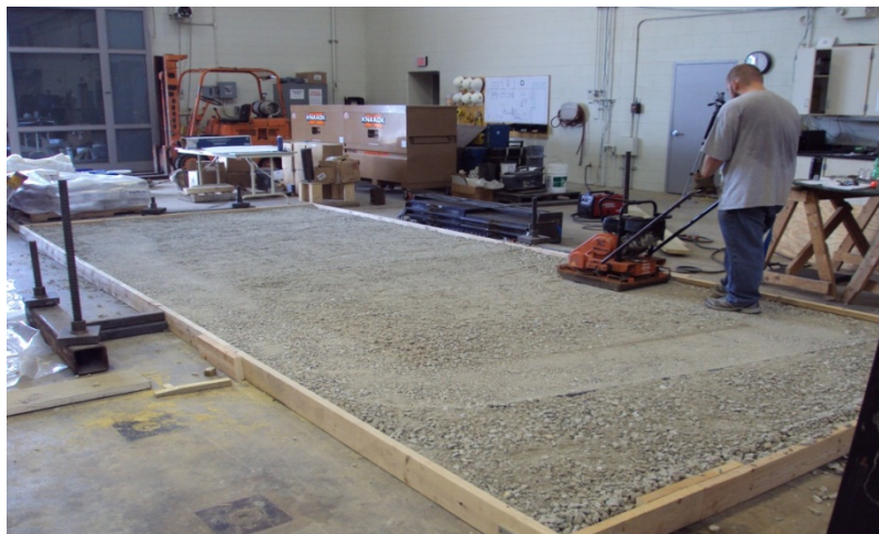
Figure 7-8 Base Material Compaction
