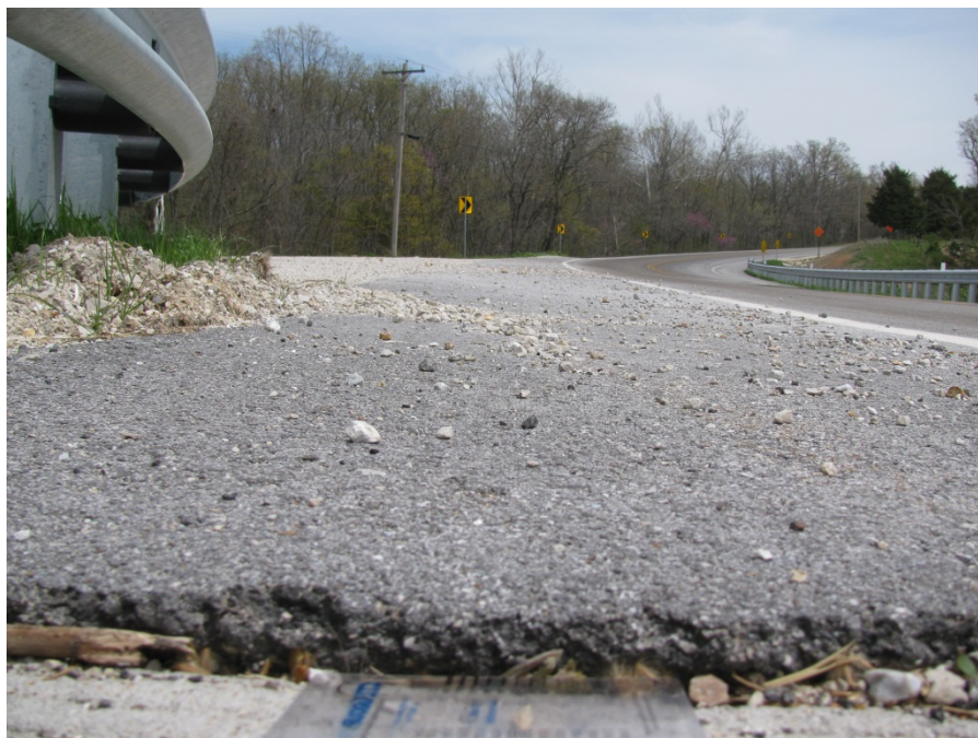
Figure 6-46 Shoulder asphalt level above the CIP BAS on MO38
