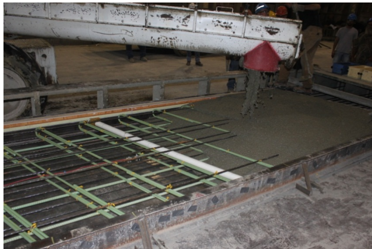
Figure 3-16 Marking of gauge location on formwork to prevent damage
