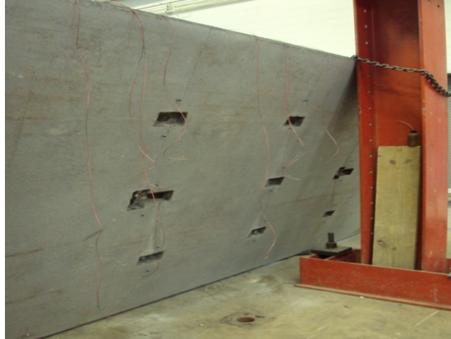
Figure 7-14 Exposure of Box Outs on the Bottom of the Panel
