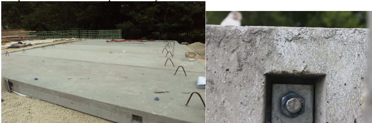
Figure 4-9 Picture showing the recesses for transverse tie rods (left) and the tie rod placed in the slabs (right)
