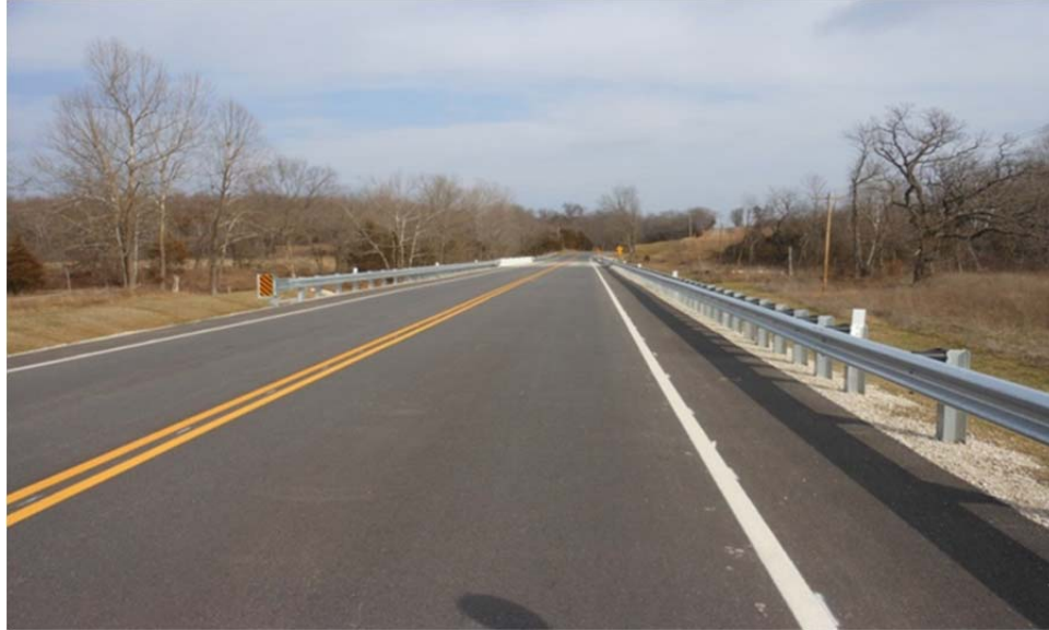
Figure 4-2 Bridge 7767 located on MO38 in Webster County, MO
